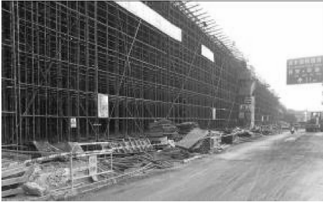
图 2 辛家庙立交桥碗扣架现场搭设情况 Fig. 2 Cuplock scaffolding in Xinjiamiao overpass construction
