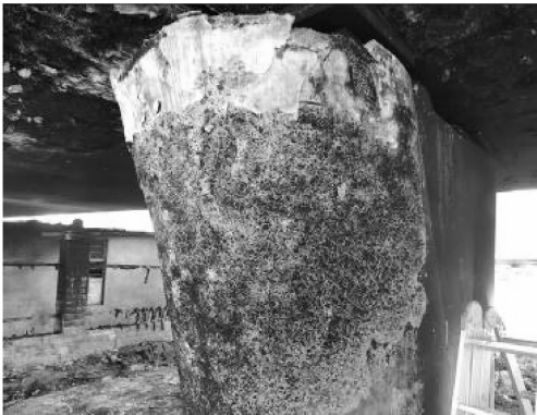
图 10 墩柱结构混凝土表面灰白色、显浅黄 Fig. 10 Pier column structure concrete surface gray white and light yellow
